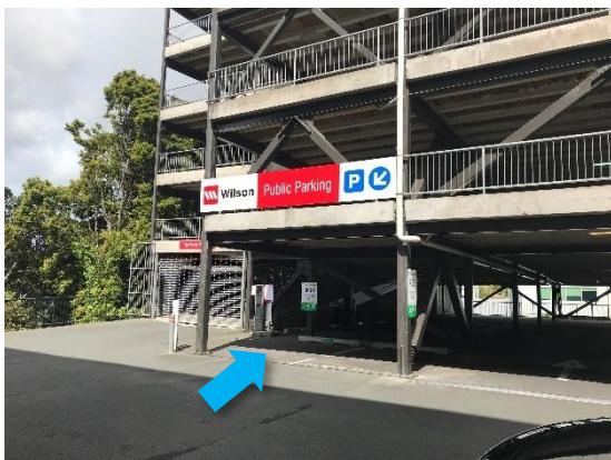
Entrance to parking building
